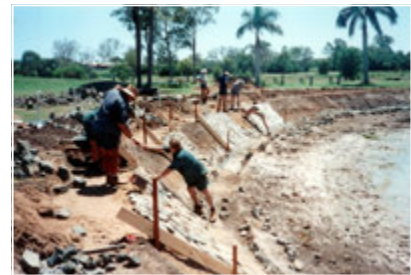
bun01835 Laying stone
