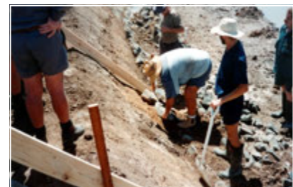
bun01832 Beginning stone bays
