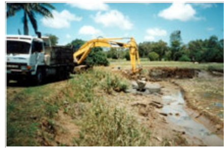
bun01831 Excavating basin in 1995
