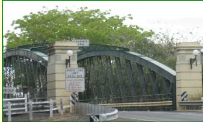
Kennedy Bridge, Bundaberg, looking to the west. 31 Oct 2010 Photo: P. Browne
