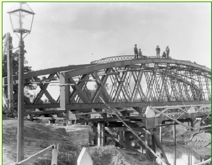
Construction of Kennedy Bridge, Bundaberg, 1898. Picture Bundaberg Collection: bun01087
