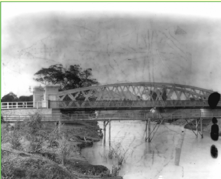
The new (1899) Kennedy Bridge and the old (1878) Kennedy Bridge, side-by-side, 1899.
