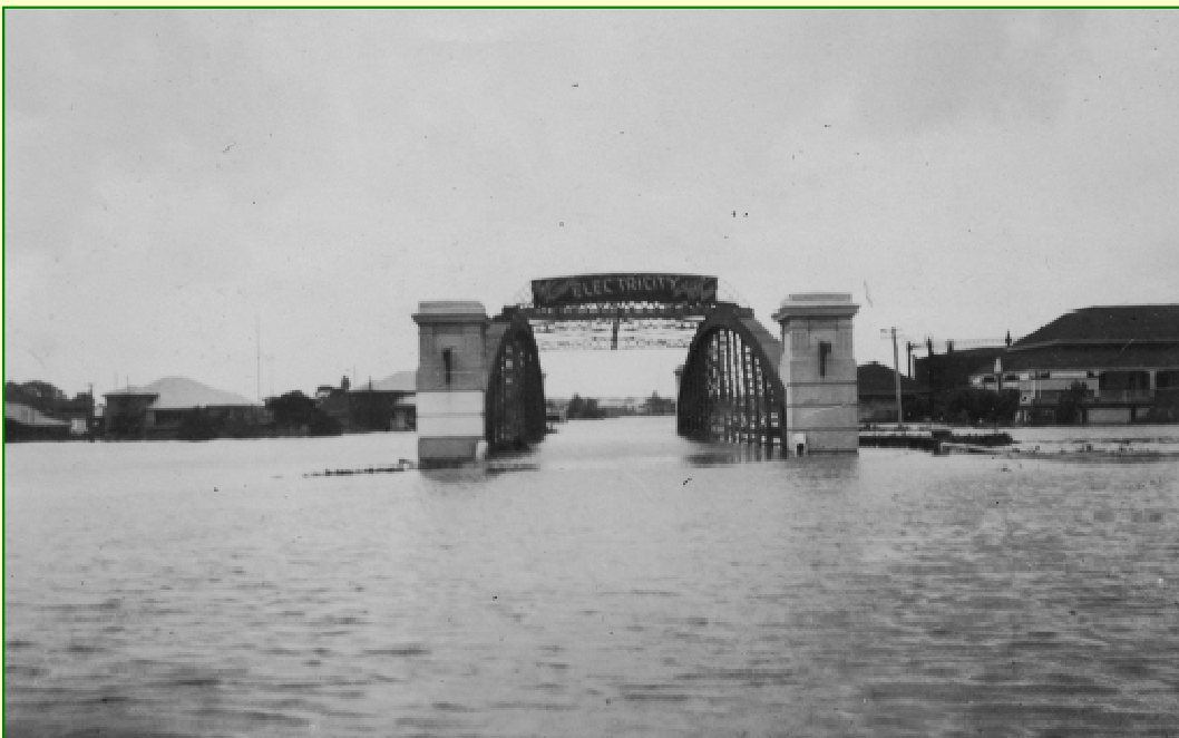
1942 floods - Kennedy Bridge.
